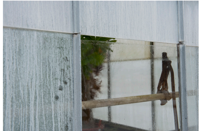
The greenhouse windows regularly fall out and require replacement due to the buckling building.
