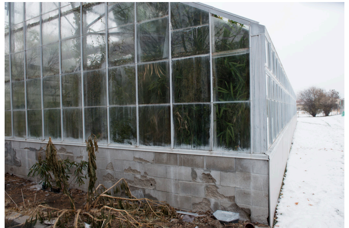
The building's insulation is threatened by a deteriorating foundation.
