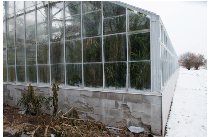
The building's insulation is threatened by a deteriorating foundation.
