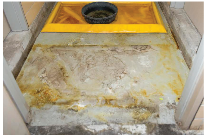
Corroded floor: Building surfaces are deteriorating and cannot withstand proper sanitation.
